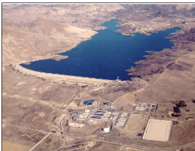
An aerial view of Lake Skinner and the water filtration facility
