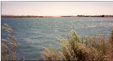
The Riverside County Municipal Dam
