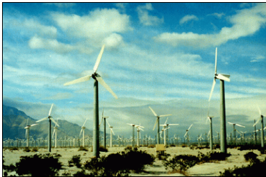
Wind turbines located in the Pass and Coachella Valley
